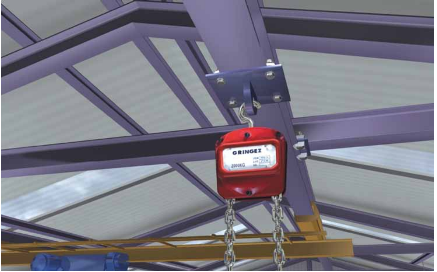
Installation of lifting equipment
